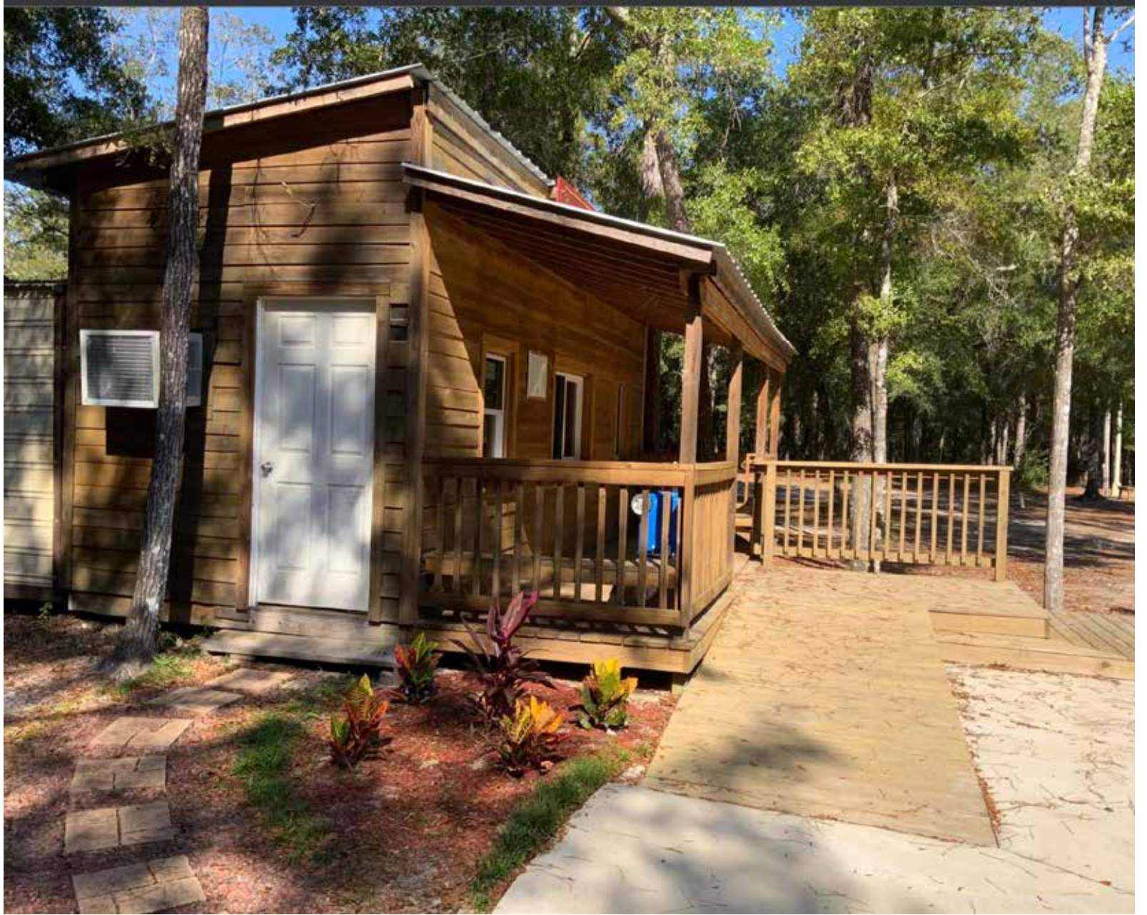
Nice pavers to the back door of the Country Store.
