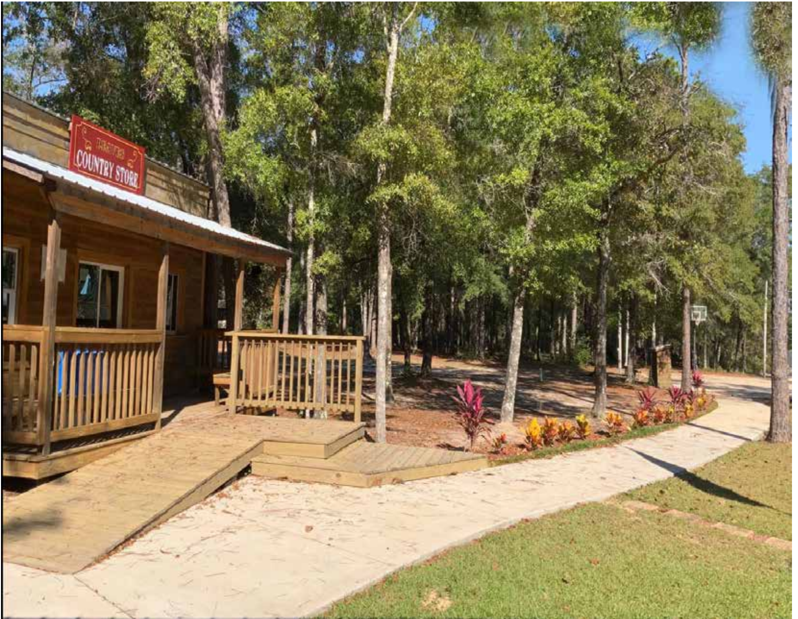
Main sidewalk from the Dining Hall to the Pool.
