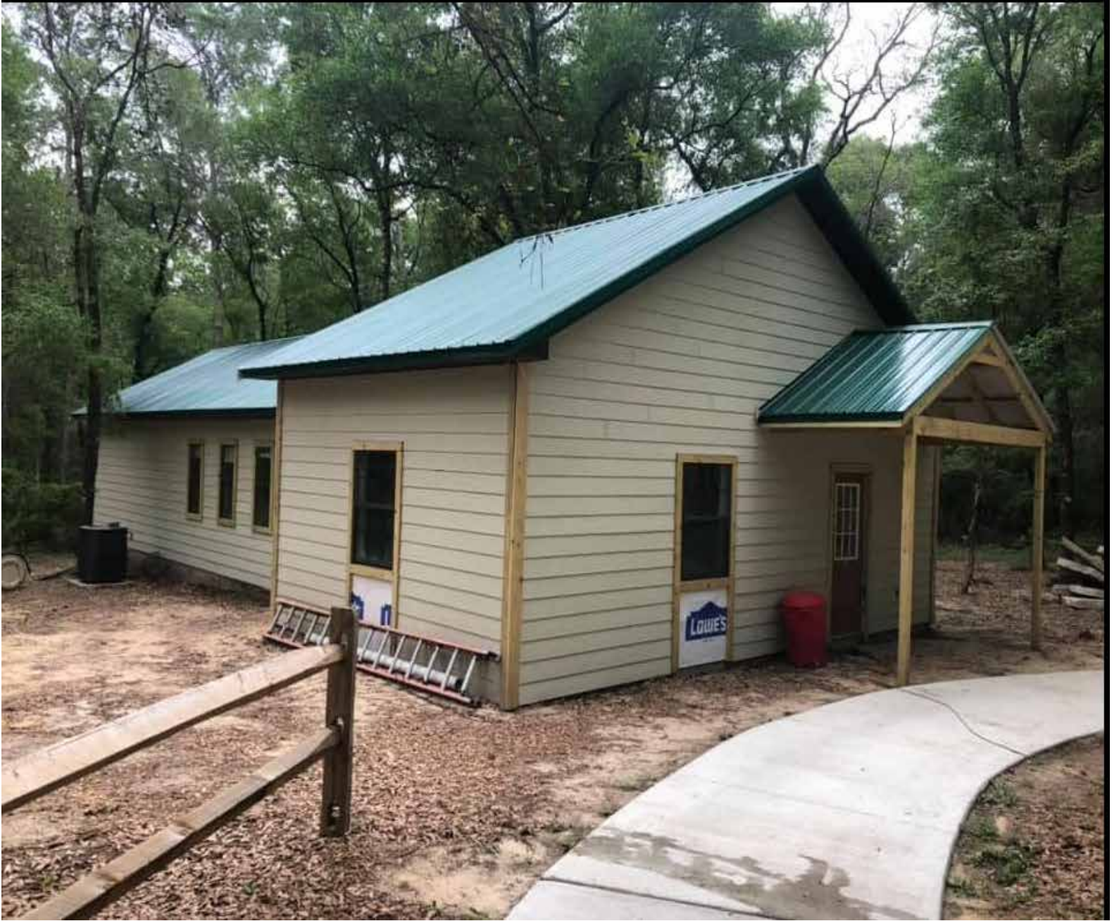
One of the 3 men's dorms is now remodeled for Handicapped Access.
